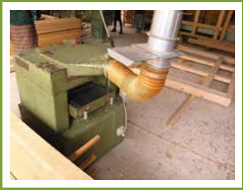
Suction port at wood working machine
