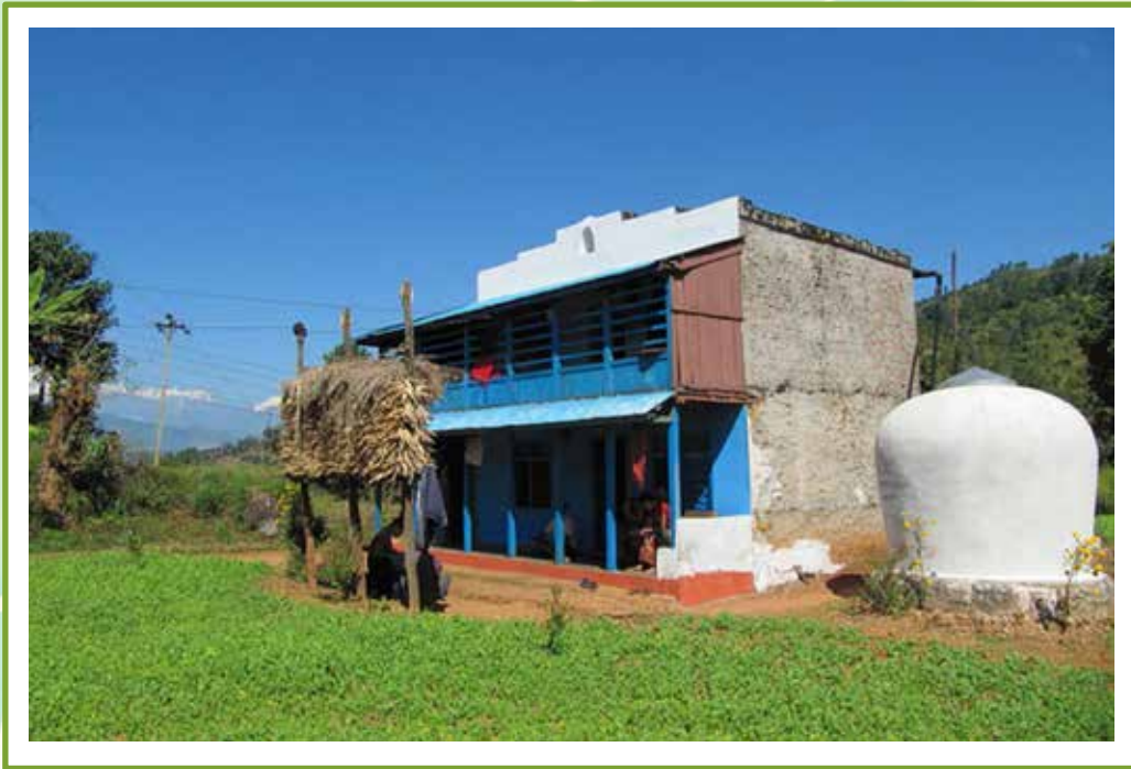
Rainwater harvesting from a shed roof via a pipe into a water tank
