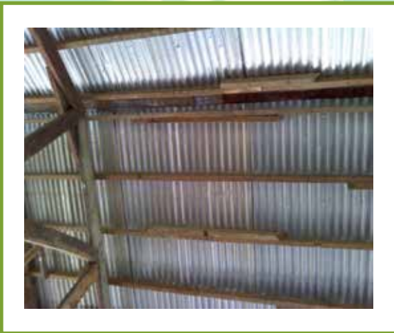
Corrugated steel roof from inside the building
