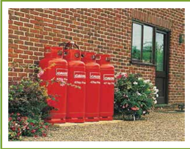
Proper storage of gas cylinders secured to a wall or inside a metal cage
