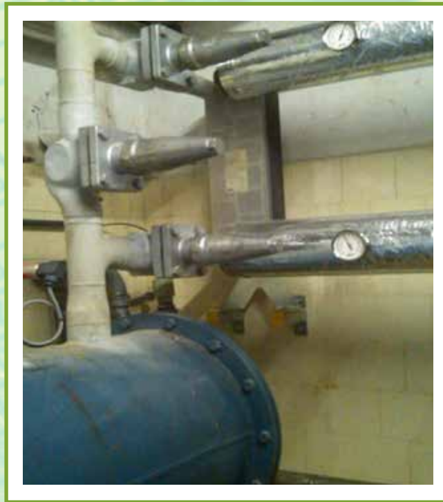
Plate type desuperheater recovers heat from hot refrigerant to heat water
