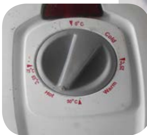
Geyser thermostat set to 55°C
