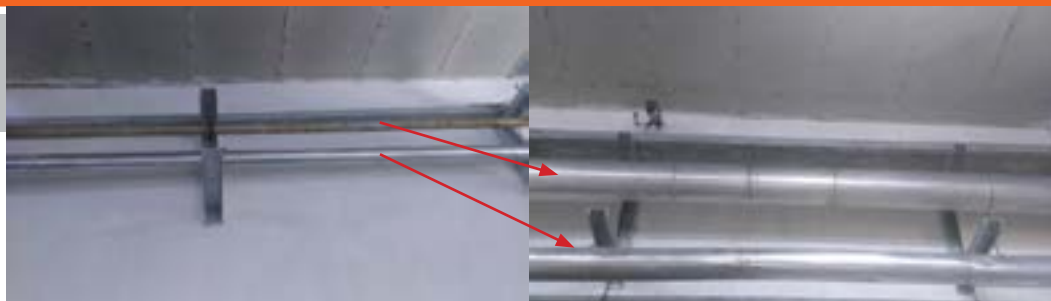
Insulation of the steam pipelines
