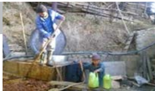
Harvesting rainwater from the weepholes in a retaining wall
