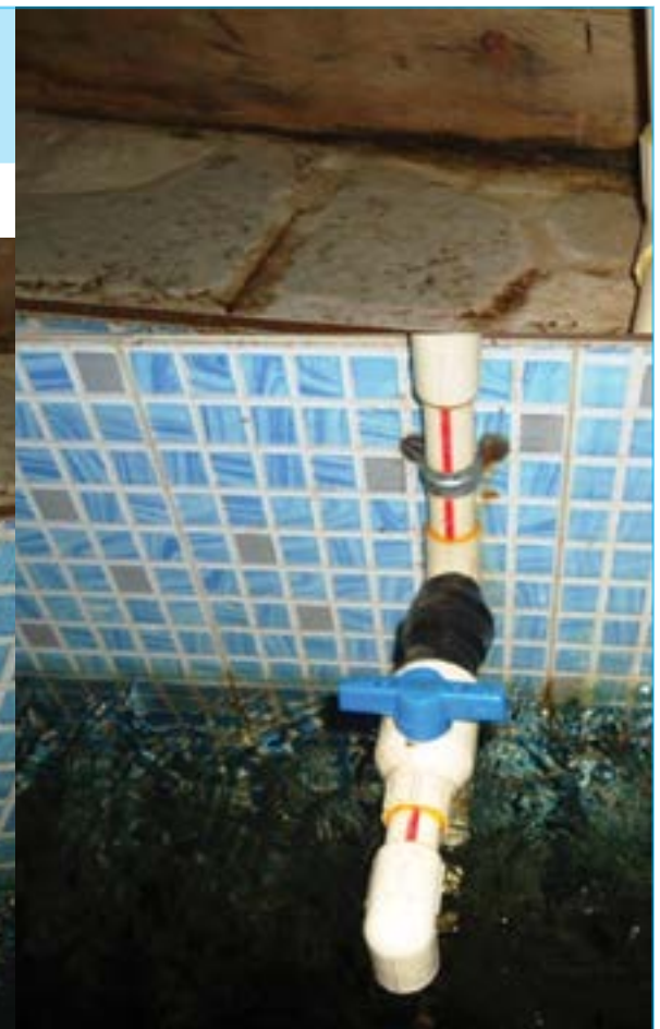
After installation of water tap
