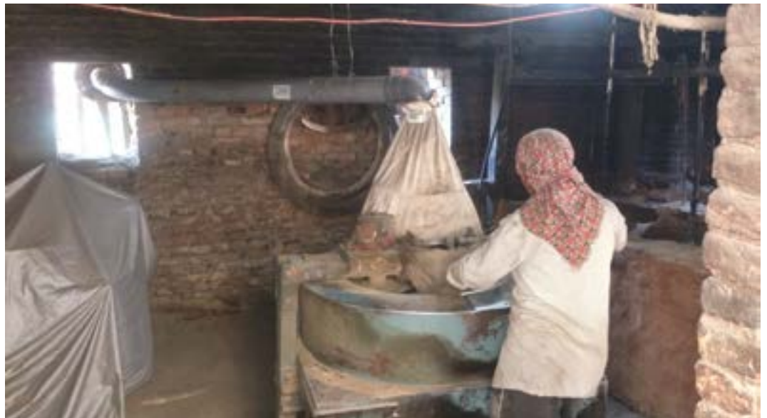
Present status: improved working environment with less dust after installation of dust collector
