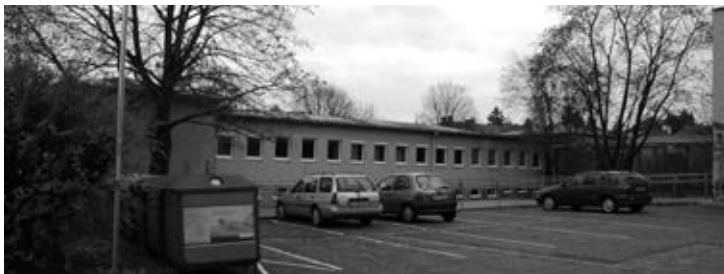
The school before renovation
